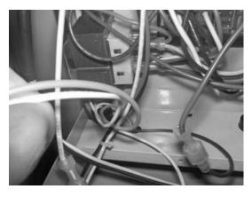
Step 12: Disconnect Pilot wires from control board and remove from Control Box
